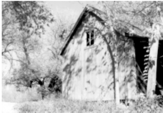
Shed to be refurbished. Photo by Tawnya Ernst
